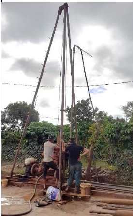
Fig. 10. The new water well Thanh-Nhan after drilling 1300m deep at IA Hét tribal village.
